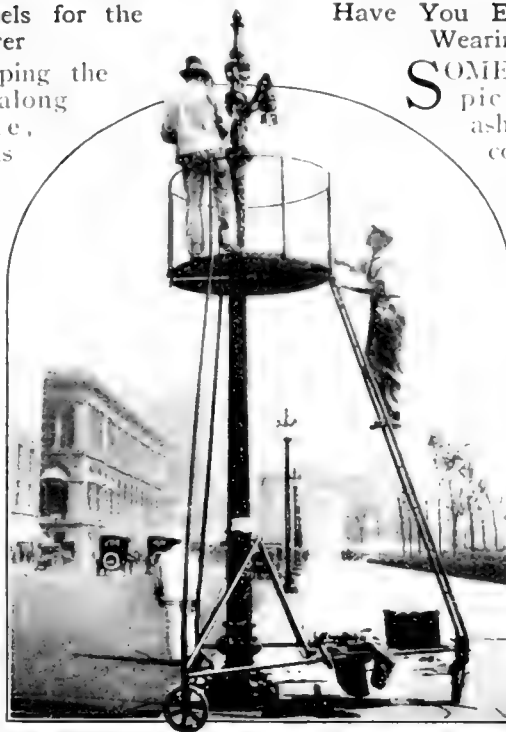
A groove is provided in the center of the platform into which the lamp-post fits closely
